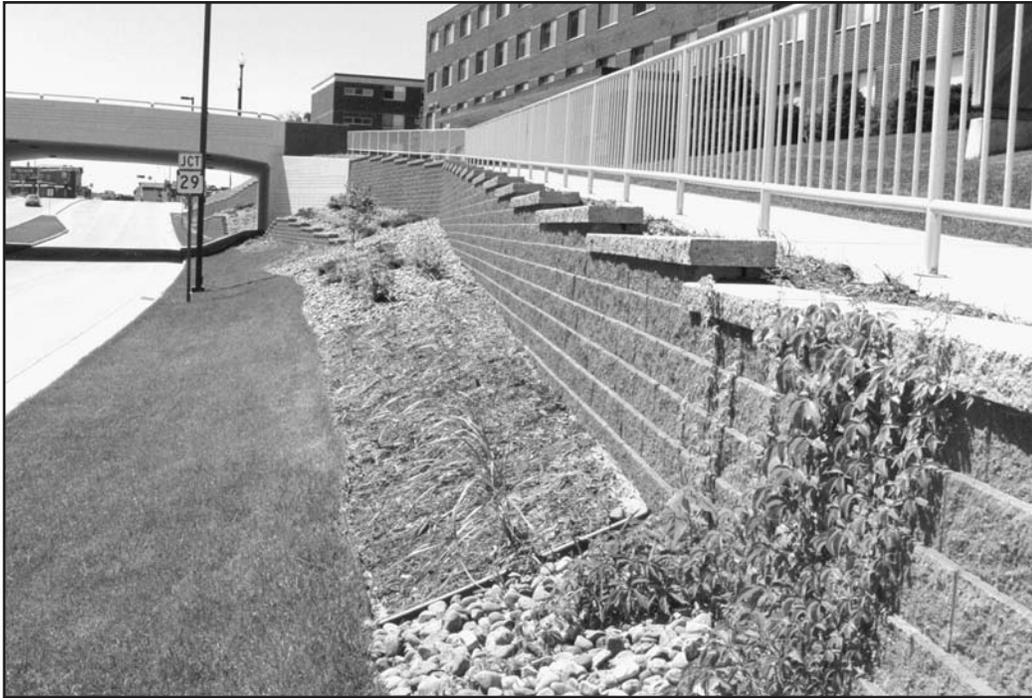
VERSA-LOK® Caps provide an easy-to-install, attractive finishing touch to the top of VERSA-LOK® Retaining Walls. Like VERSA-LOK wall units, VERSA-LOK Cap units are solid. The cap units also have textured split-faces and colors that match retaining wall units.
