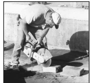
Saw-cutting can easily be done in the field. Start by laying caps at each fixed point. Then work away from these points until the cap units nearly meet, leaving only a gap smaller than a whole cap unit. Saw-cut a partial cap unit to fit in this remaining gap. Try to keep the remaining gap towards the center of the wall. This helps hide smaller cap pieces.
